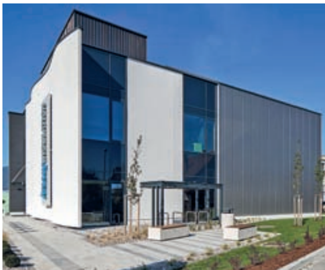
Knauf Insulation Experience Center, Škofja Loka
